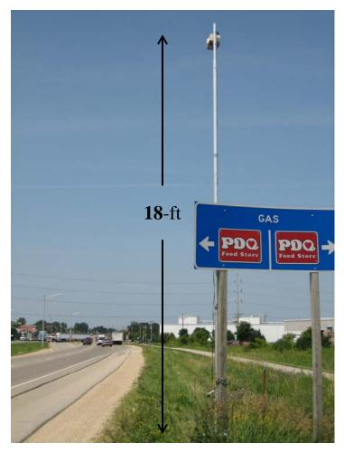
FIGURE 1 Typical video camera installation.
